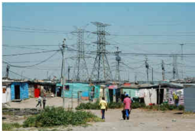
Figure 2: Joe Slovo informal settlement, showing electrification infrastructure
